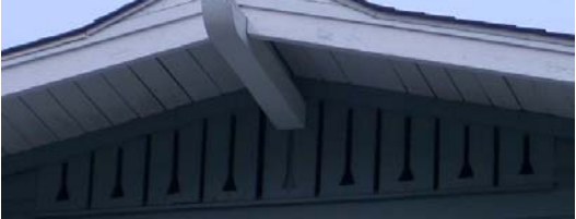
Vertical Slat Vent w/Decorative Cut Outs:
