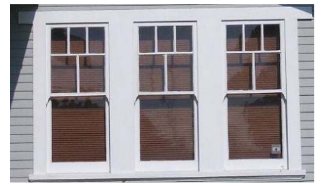
Ribbon (triple) wood cased double hung windows with five geometric lights over one light and an extended lintel.
