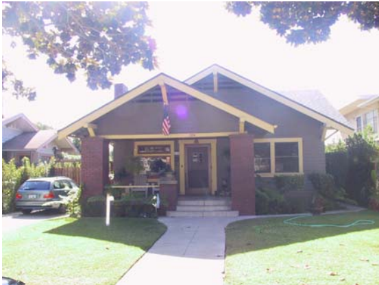
Front Gabled Roof
