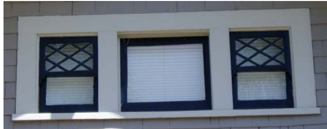
Two wood cased casement windows with diamond-patterned multi-light designs flanking one single pane wood cased fixed window with wide wood surrounds.
