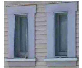
Two small narrow wood cased casement windows with wide wood surrounds.
