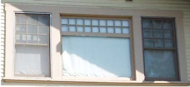
Two wood sash double hung windows with nine lights over one light flanking one large fixed window with 18 multi-lights surrounded by a wide wood surround.
