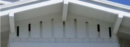
Picket Fence Vertical Slat Vent:
