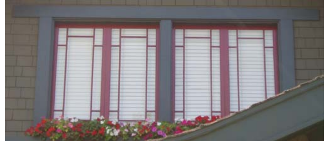
Set of ribbon windows (likely two sets of paired casements) with Craftsman-style geometric mullion design and extended lintel.
