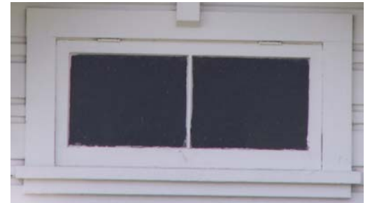
One wood cased awning style window with two lights and wide window surrounds.
