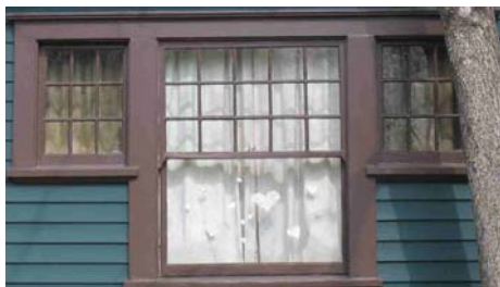
Two wood cased fixed nine light windows flanking one large double hung window with 15 lights over one single wood sash.
