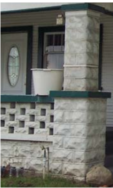
Ornamental Concrete Block Columns and Pedestals:
