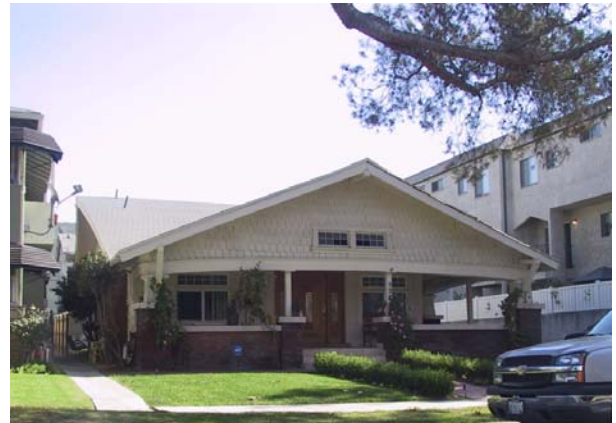
Cross Gabled Roof
