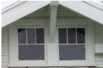
Paired wood cased casement windows with three narrow rectangular lights over one horizontal light, each cased in wide wood surrounds.
