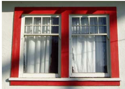
Paired wood cased single hung windows with 8 small lights over one single pane and wide wood surrounds.
