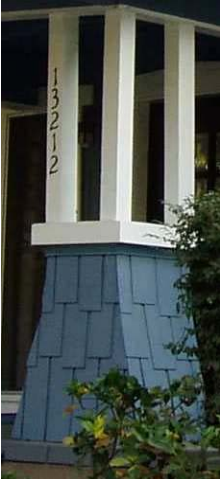
Wood Shingled Pedestals:
