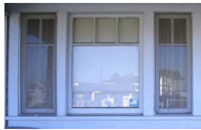
Two wood cased casement windows with two small lights over one vertical light flanking one fixed window with three lights over one light with a wide wood surrounds.
