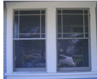
Paired wood cased double hung windows with Craftsman mullion design over a single pane.
